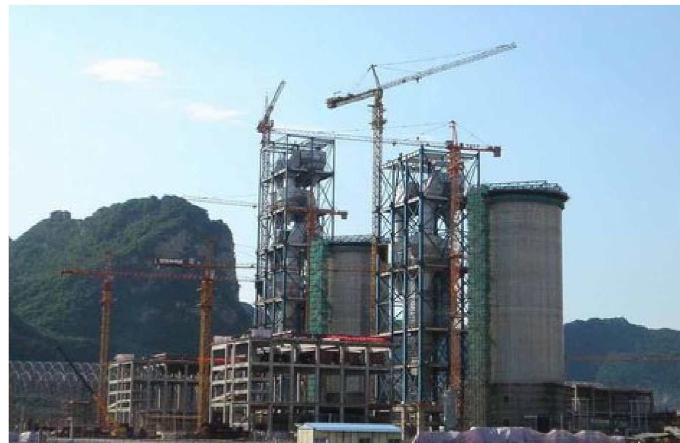
广州金关公司开展的台泥（英德）有限公司的水泥熟料生产线大型风机变频节能技术改造工程 Guangzhou G.K. Energy Services Co., Ltd installed variable frequency drives on a large fan system in the Cement Clinker Production Line of TCC (Yingde) Co., Ltd.
